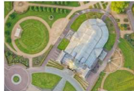
Glasgow plans £36m overhaul of People's Palace
